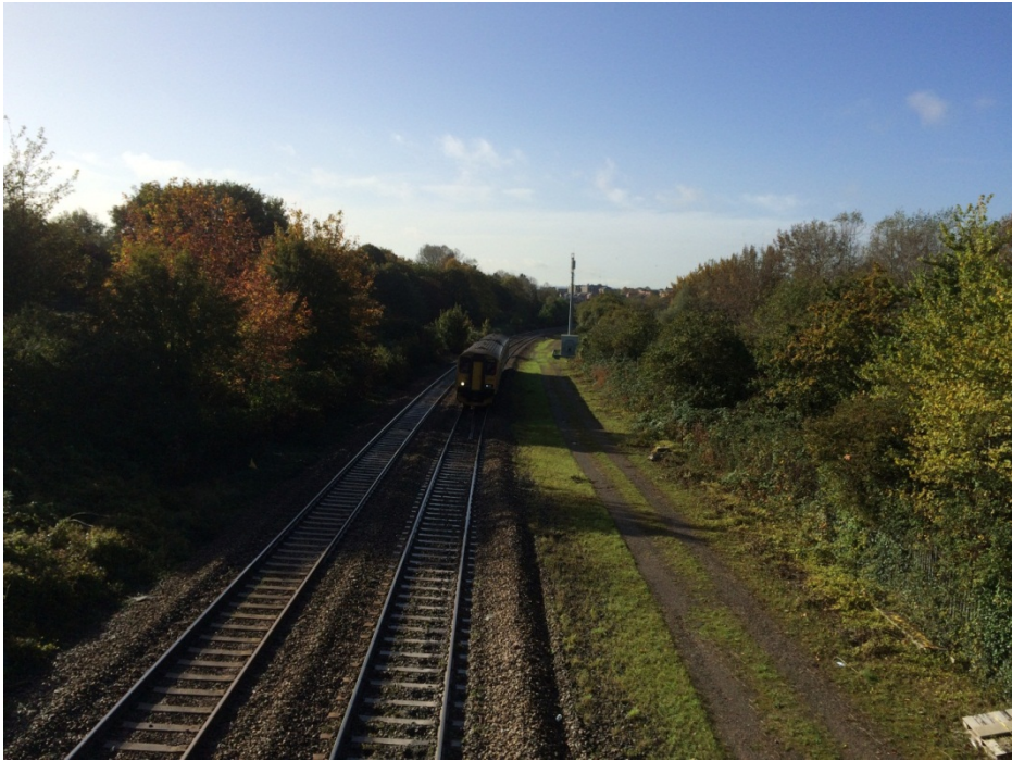
Photograph 7: Filton Bank looking south towards Bristol Temple Meads
