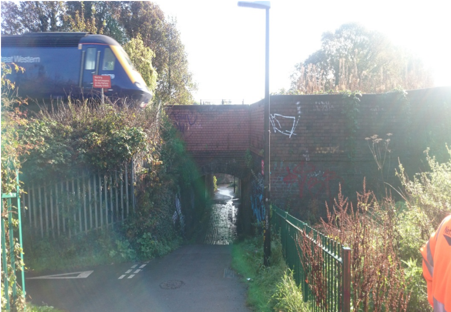
Photograph 4: Footpath underbridge at proposed station location (West portal)
