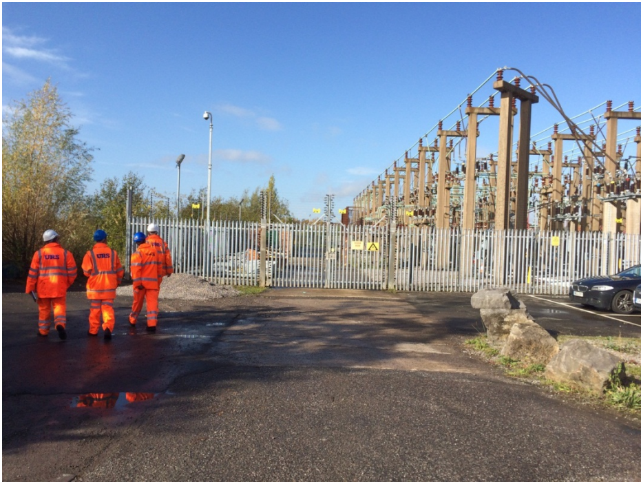
Photograph 13: Substation adjacent to Filton Bank proposed station (Constable Road Site)
