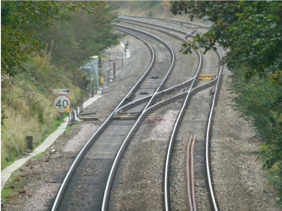
Photograph 28: Turnouts near Yate station towards Westerleigh Junction
