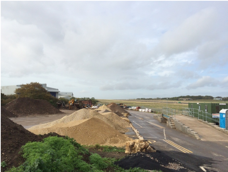
Photograph 17: Proposed location for car park and vehicle access for North Filton
