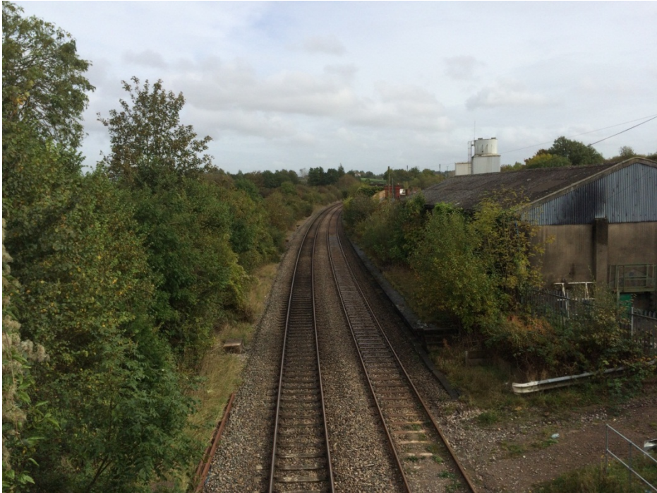
Photograph 22: Former Henbury station platform looking towards East
