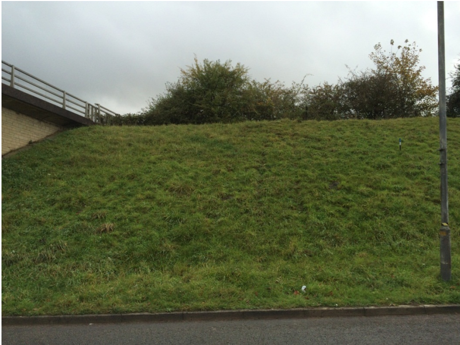
Photograph 18: Proposed pedestrian access on top of the embankment
