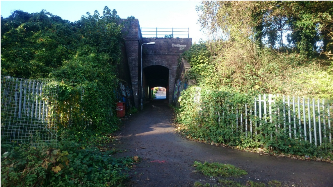
Photograph 6: Footpath underbridge at proposed station location (East portal)
