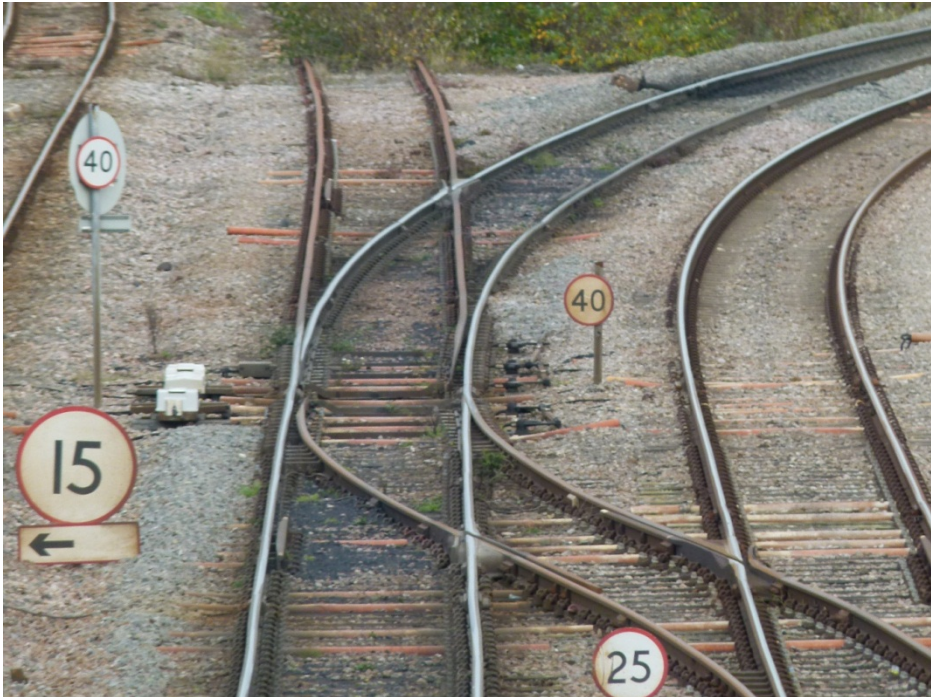
Photograph 24: Turn outs at Hallen Marsh Junction
