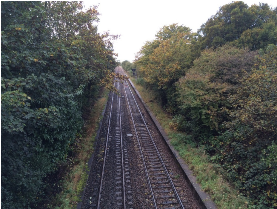
Photograph 15: North Filton (looking West towards Henbury)
