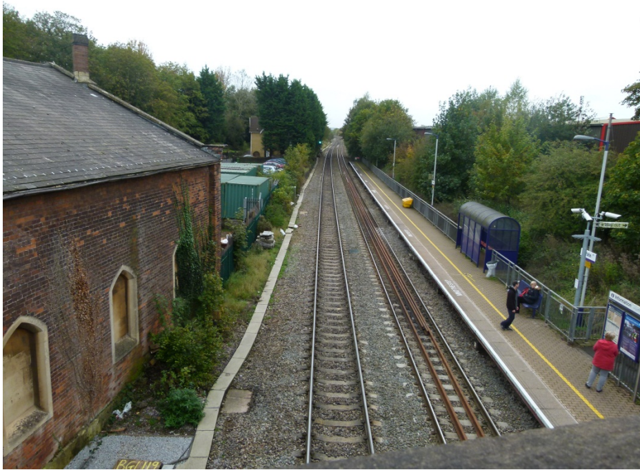
Photograph 29 Yate Station platform 1 looking south towards Westerleigh junction
