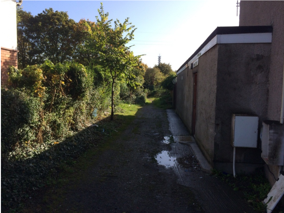
Photograph 9: Pedestrian access to existing footbridge from west side of the railway (Dover Court Road)
