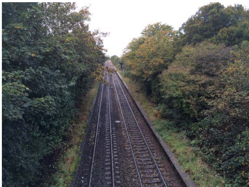
The existing Freight Route – Filton West Junction to Hallen Marsh Junction and the redundant platforms at North Filton
