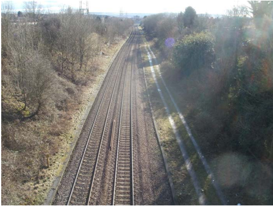
Figure 2-14: Existing 2-track layout showing Horfield future station location (looking south from Bonnington Walk)
