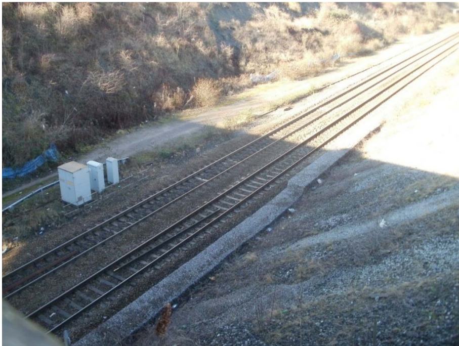
Figure 2-15: Cutting slope to the north of Bonnington Walk bridge
