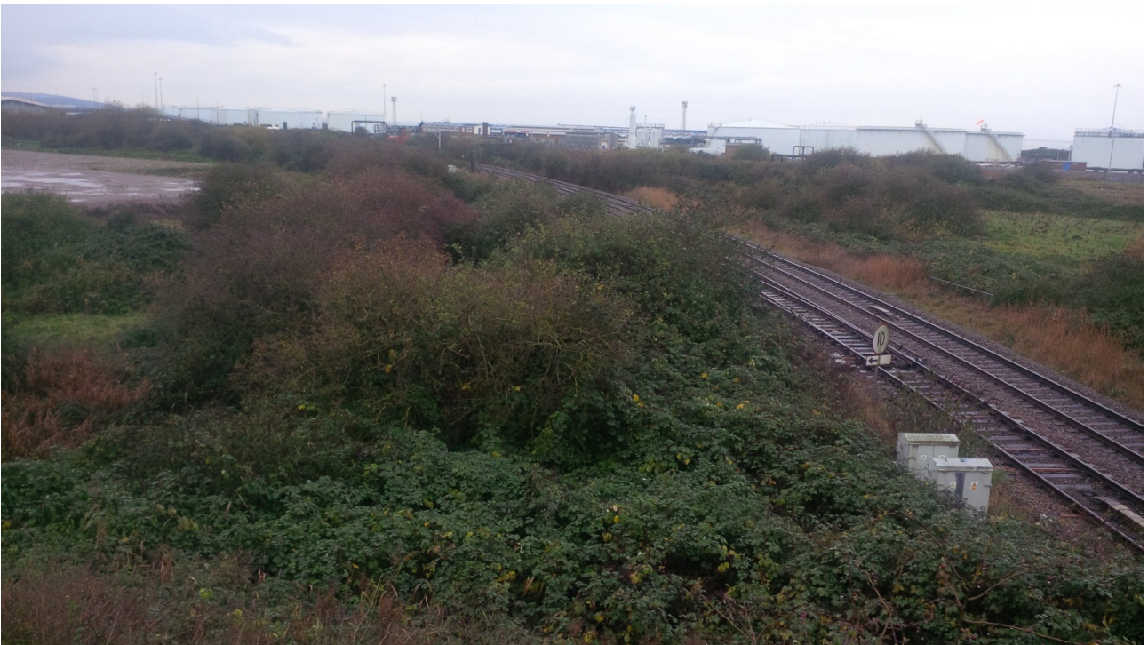
Photograph 8.2: View from Smoke Lane Bridge, possible access from the left. Vegetation to be cleared.
