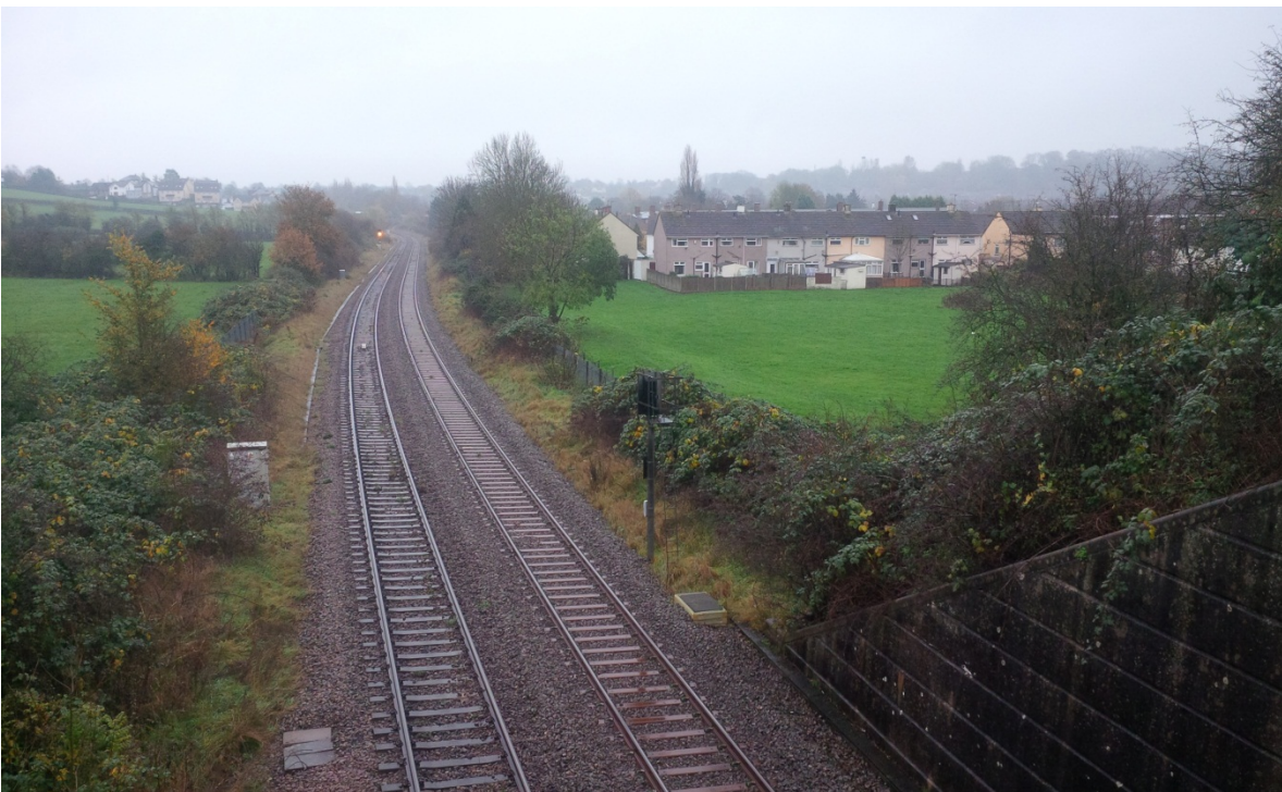
Photograph 8.3: View from A4018 bridge over the existing line. Open space and houses to the right.
