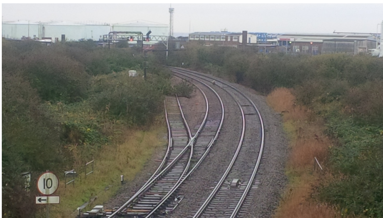
Photograph 8.1: View from Smoke Lane Bridge to junction.
