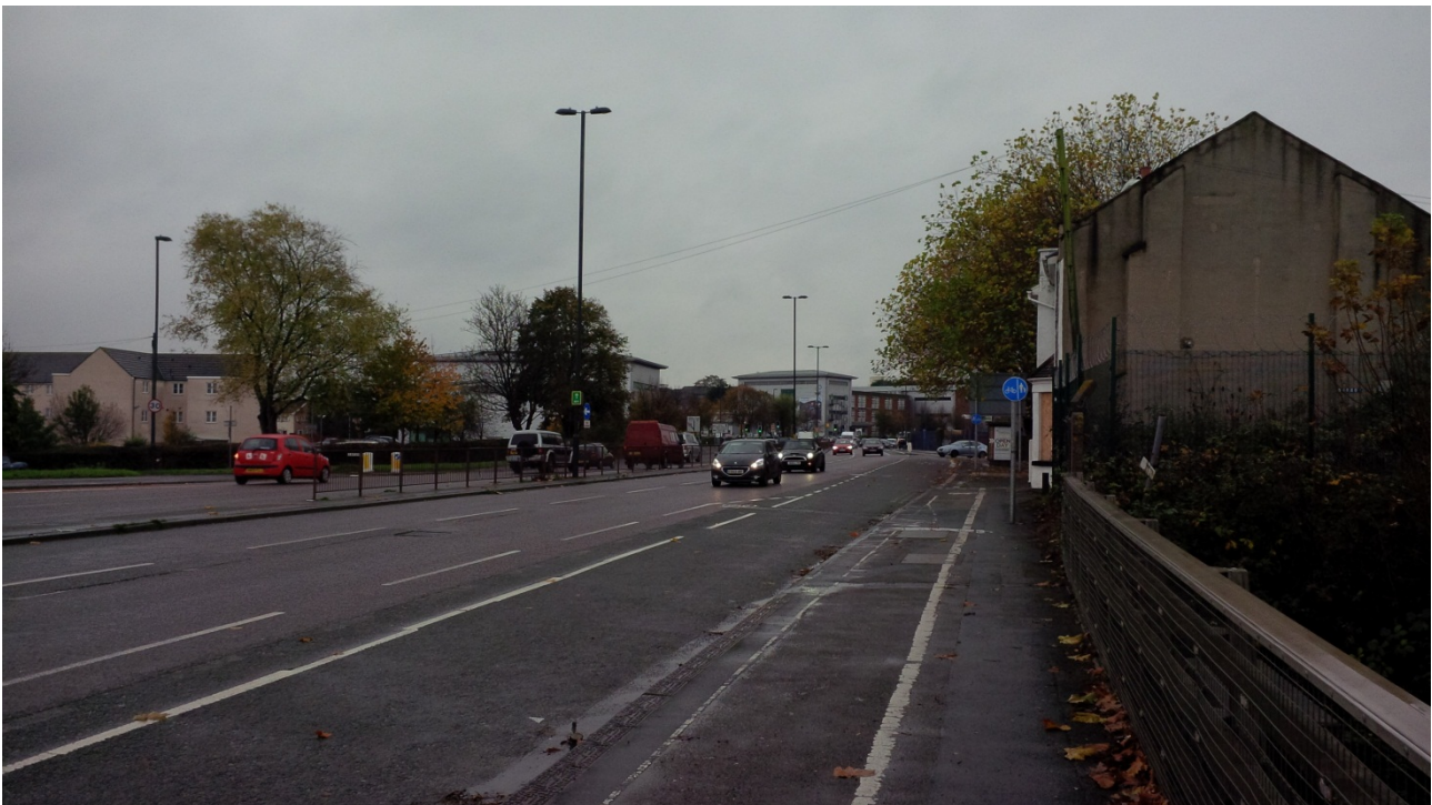
Photograph 8.3: Looking south on A38 Gloucester Road (dual carriageway), building to be demolished on right, residences on left.
