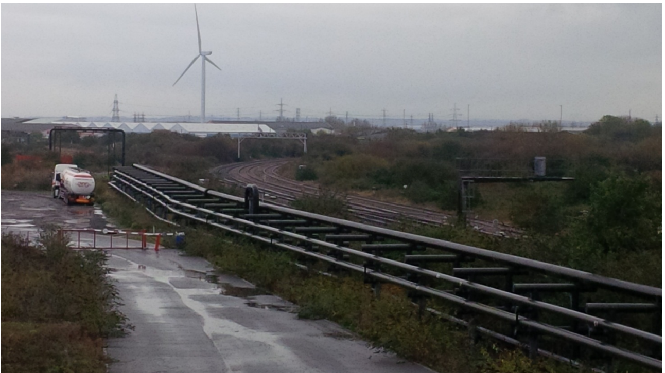
Photograph 8.2: View NE from port access road bridge, off St Andrew's Rd.
