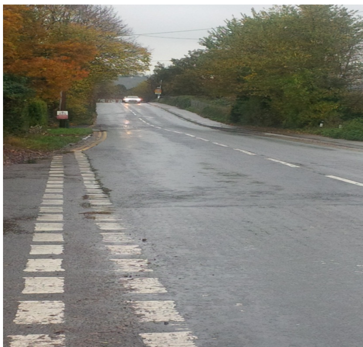
Photograph 8.3: Looking south to station road bridge
