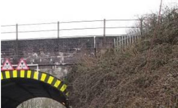
Displaced Parapet
