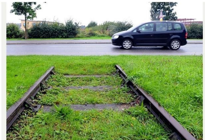
Trains will be running out of Portishead again by 2019
