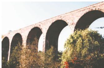
Railway Viaduct at Pensford
